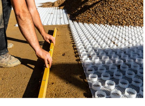
The added benefits of using Graveledge alongside Gravelrings does not come at the expense of a tricky installation. Graveledge edging can simply be installed around the perimeter of the gravel driveway with a dry fix installation, meaning no concrete is required. Even better, Grave-
